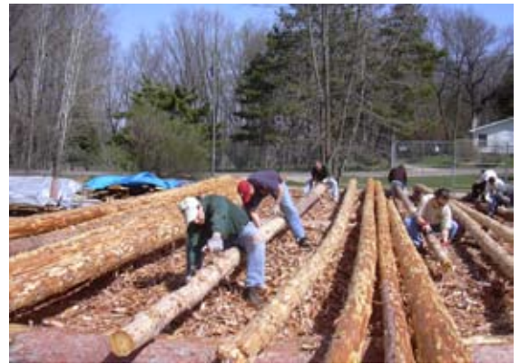
Volunteers peel logs at the building site
